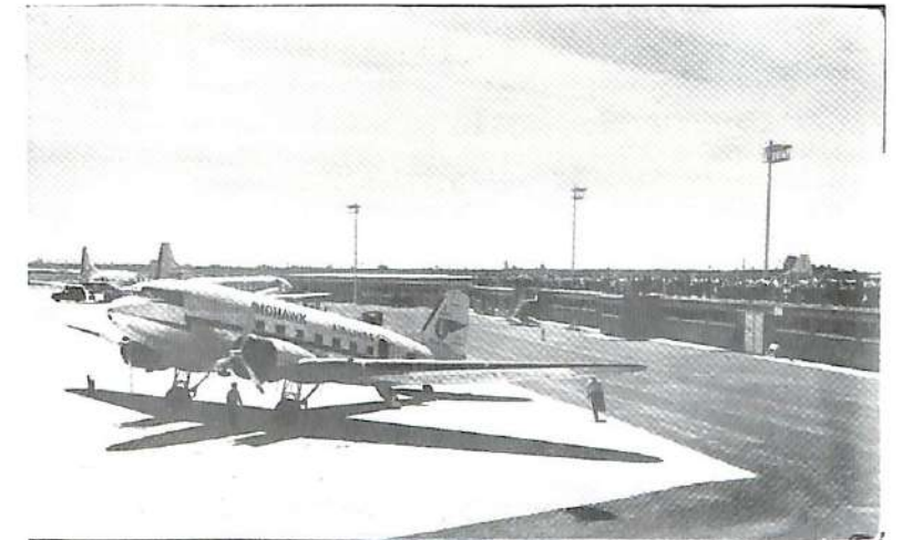
VW Observation deck and plane ramps at Newark Airport. Photo courtesy of The Port of New York Authority.
