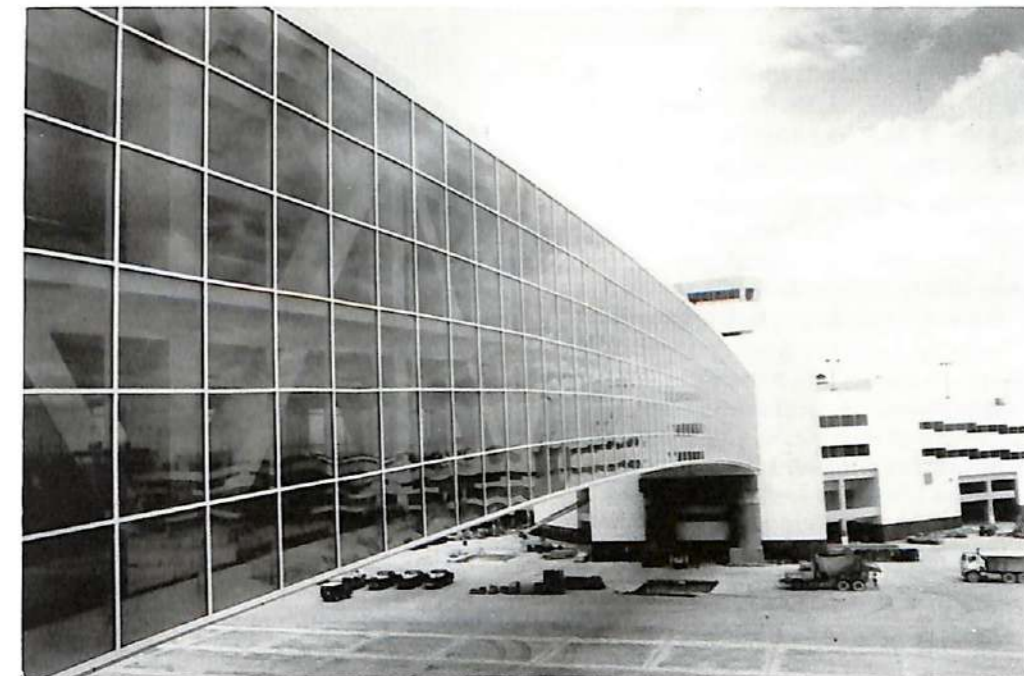
Passenger bridge between the main terminal and Concourse A is high enough to let 737s taxi underneath. (All photos by the author.)
