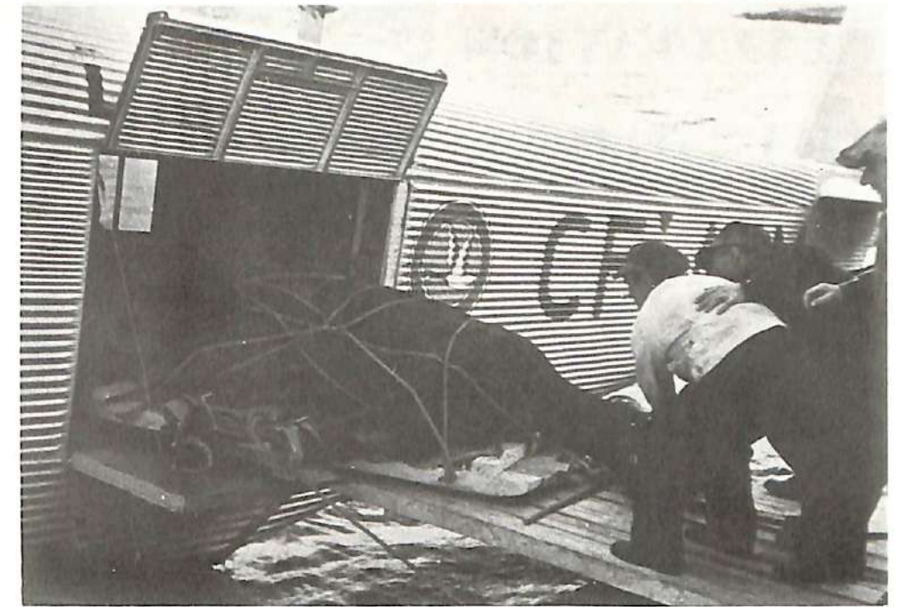
A DRUGGED HORSE IS SKIDDED ABOARD THE JU 52 CF-ARM OF CANADIAN AIRWAYS ON A SPECIAL LOADING RAMP. WITH THE JUNKERS BEING THE LARGEST AIRCRAFT IN CANADA AT THE TIME, A SPECIAL LOADING DICK HAD TO BE BUILT FIRST WHEREVER SHE WENT TO PICK UP PASSENGERS OR CARGO. ON ONE TRIP IN 1932, 10 PROSPECTORS, FIVE CAMOES, FREIGHT AND THREE CREW WERE ON BOARD. (Photo courtesy Western Canada Aviation Museum)
