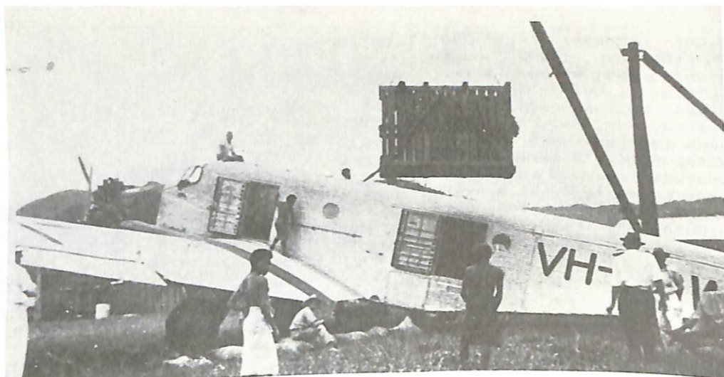
Above: Junkers G31 VH-UOW of Guinea Airways being loaded with heavy equipment for delivery inland on New Guinea.
