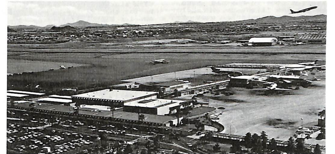
TOP: Land side of Sky Harbor's curved Terminal 1 shortly after World War 2. Note the DC-3 nose to the left of the building. ABOVE: 1976 photo of Sky Harbor, showing Terminal 2. Terminal 1 is just outside this photo to the right.
