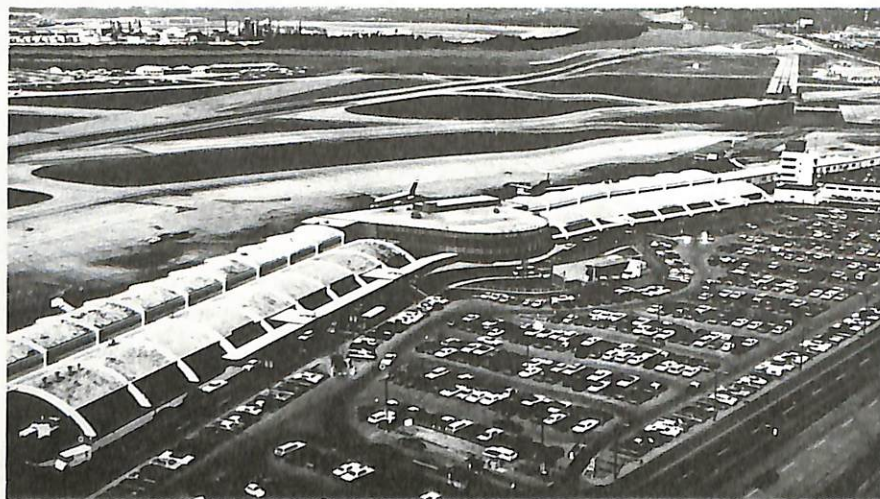
MCI, Kansas City International. View to the north shows terminal A in left background, B and C left and right foreground. Terminals can handle 10-12 million passengers per year. 10,800 ft (3,300 m) N/S main runway is at upper left. Second runway runs E/W and is 9,500 ft (2,900 m). Land for fourth terminal has been reserved in right background. ATC tower in center is also shown in photo of restored Northrop Alpha with this history.
