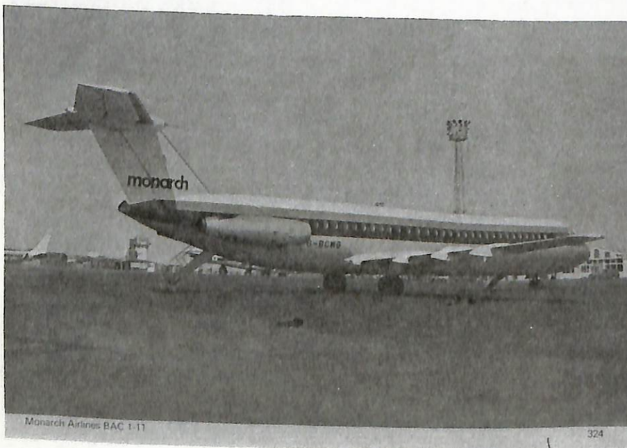
This post card of a Monarch BAC One-Eleven gives a good view of the T-tail that caused major problems on the prototype aircraft.
