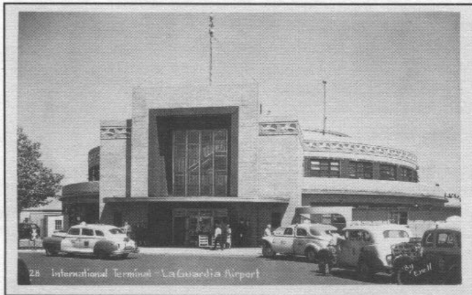
Front of Marine Air Terminal (International Terminal), 1940s. Enell no. 28. B&W.
