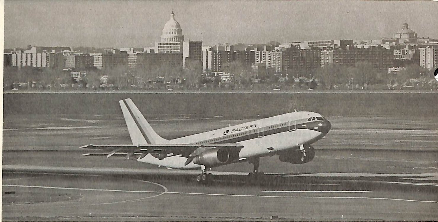
The first landing ever by a wide-body airliner at Washington National Airport when this Eastern Airlines A-300B4 visited the capital's airport at the invitation of the Federal Aviation Administration. The big jet performed a number of noise measurement flights which proved it to be much quieter than the smaller jets currently using the airport. Photo courtesy of Eastern Airlines.
