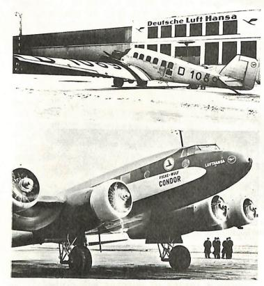
The Focke-Wulf Fw 200 Condor was the first land plane used on Lufthansa's long distance services. It was used in 1938 on a non-stop Berlin—New York flight.
