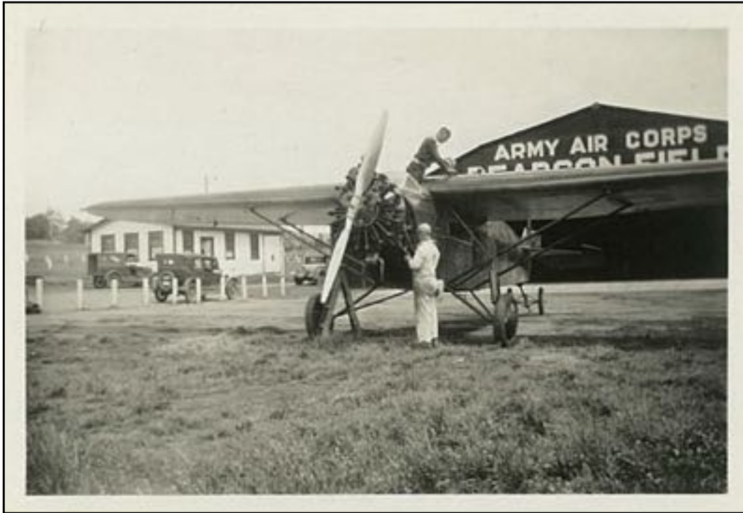
Pearson Field was home to Pacific Air Transport. The pilot of the Fokker Universal sat in an open cockpit forward of the wing's leading edge, and the enclosed cabin below and to the rear of the pilot held 4-6 passengers. Photograph copyright unknown.
